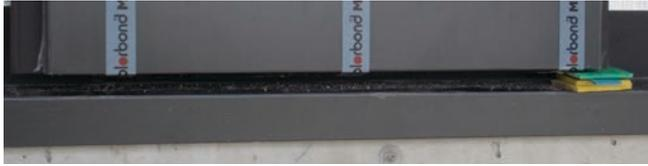
7. When installing the first panel, packers/shims may be used under the male leg to assist with engaging into the female edge, and ensure a flat plane of the finished surface.
