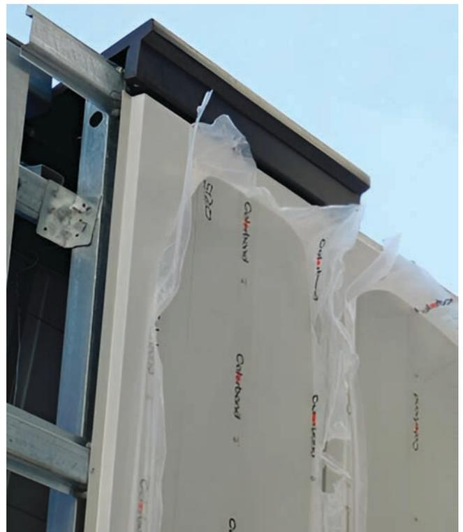
6. Temporary spacer blocks, a straight edge or stringline may be used at the panel ends to help align the panels and ensure a uniform gap at the ends of the panel.
