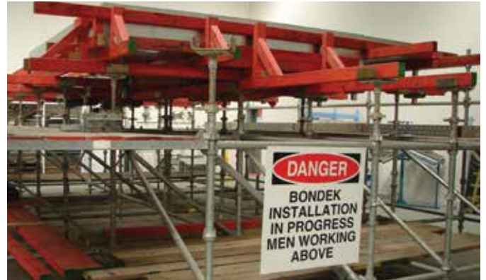
Step 2: Place props if required.
