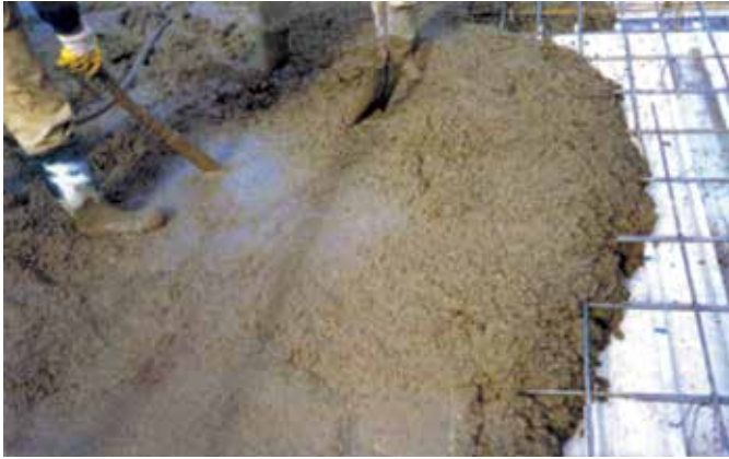
Step 8: Place concrete.
