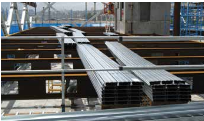
Step 3: Trim BONDEK® sheets if required and place.
