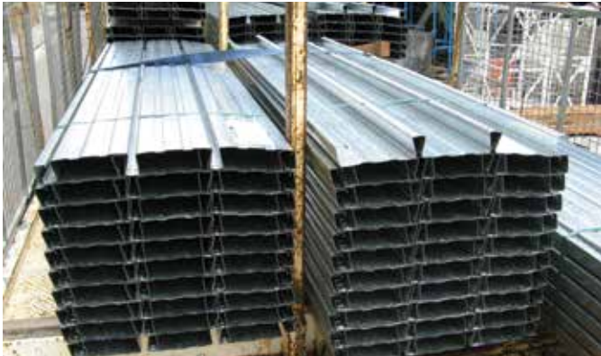
Step 1: Open BONDEK® sheet bundles.
