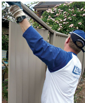
Lifting top rail helps ease 1st sheet into end position.
