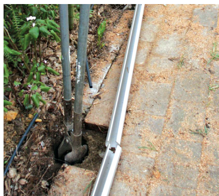
Lay the rails along the string line to determine positions of posts.
