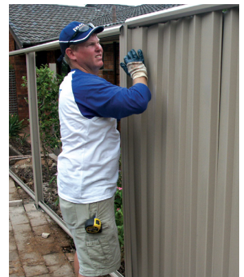
Lift top rail and rotate until infill sheet slides into rail. Tap top rail down into position.
