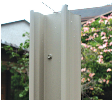
Use stringline to set post heights.
