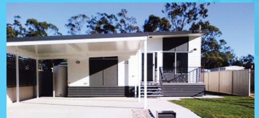
LYSAGHT Living Collection® carports at a Dysart mining community in mid 2012
