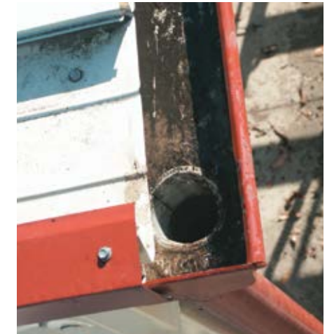
3) When litter is removed, the layer of hardened dirt is revealed below.
