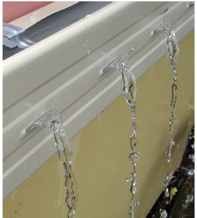
*Typical overflow from slotted gutter.*
