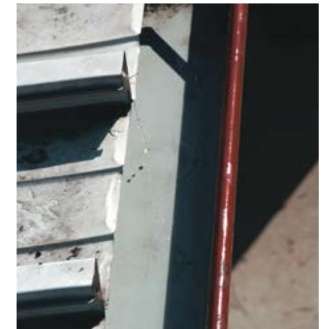
6) When the gutter has been cleaned, it should look like this.
