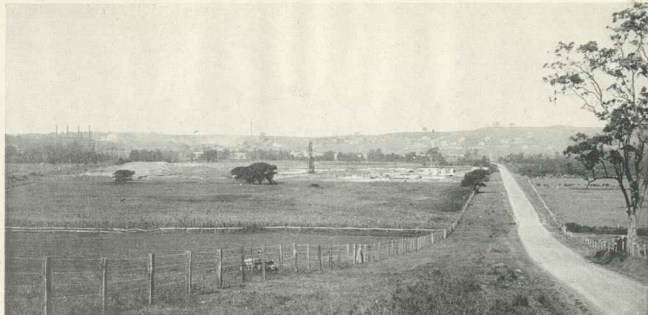
The site of Lysaght's Port Kembla Works, April, 1937, showing the pile driver at work on the foundations, and the encroachment of the filling, which was carried right across the site to the top level of the piles. Approximately 310,000 cubic yards of filling were used, raising the original ground level an average of 10 feet. The Australian Iron and Steel Works are seen in the background.
