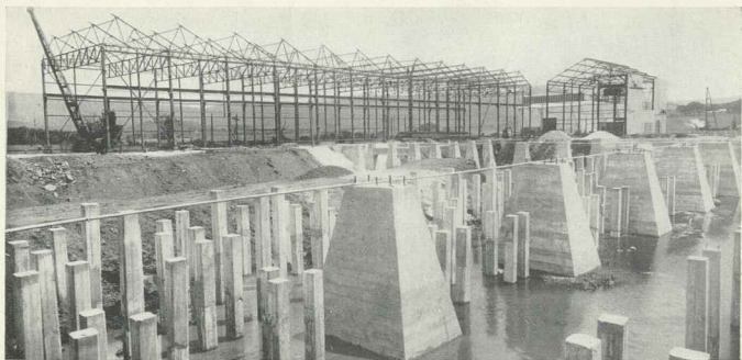
By November, 1937, indications of things to come were evident—foundations, filling and fabrication all going ahead simultaneously.
