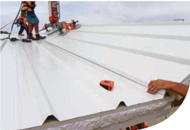
**Figure 5.4 ALSULATE-125® panels after joining**
