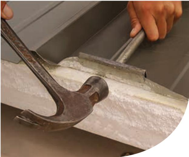
**Figure 4.4: Turn down all the roof pans at the gutter end using the turn down tool**
