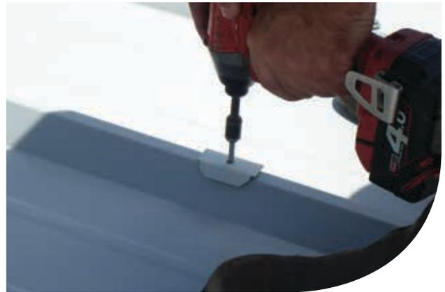
**Figure 4.6: Screw installation**
